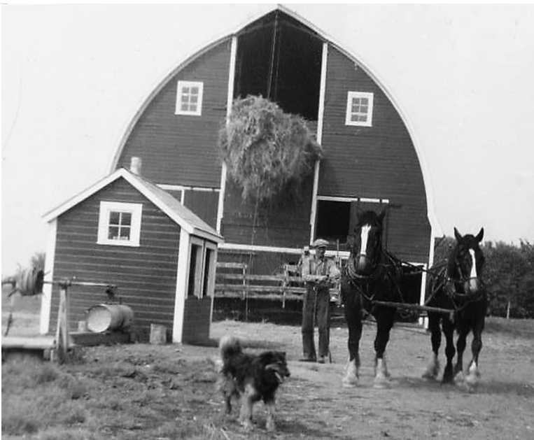
A wagon, which has been loaded with hay, is parked in front of the barn doors. The farmer has unhitched from the wagon, and has hooked on to a cable which is used to lift the hay from the wagon up into the loft of the barn.
